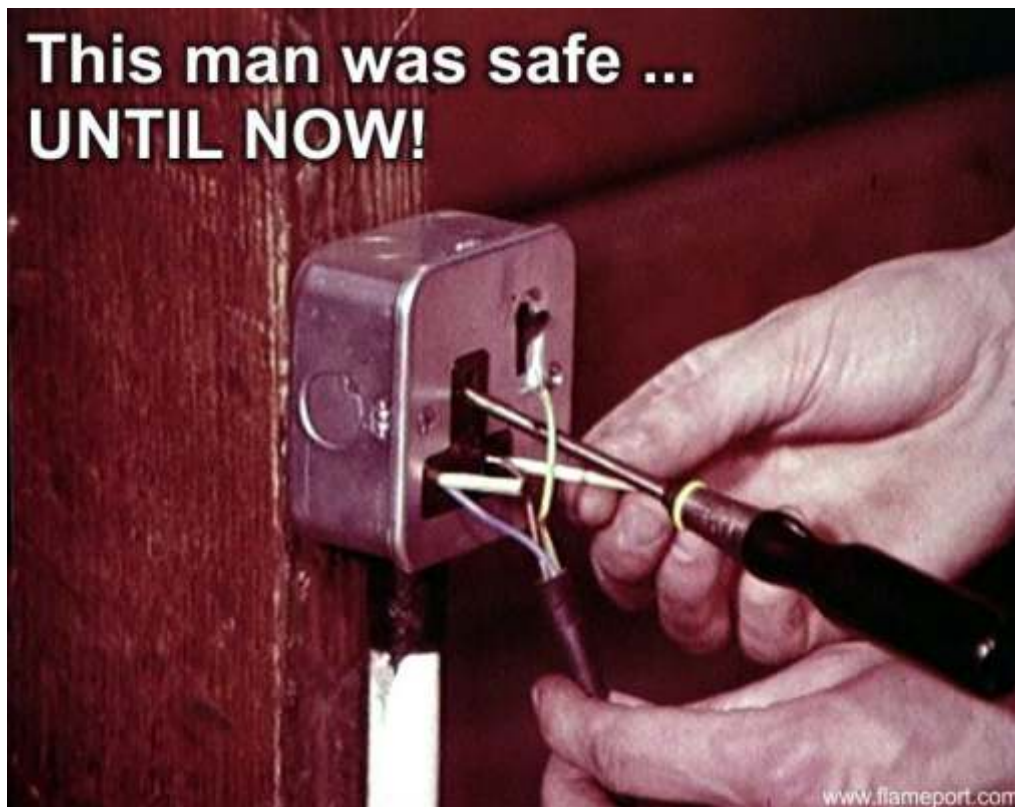
Fig 5.1.1.2: Example of a Potential Accident Area
