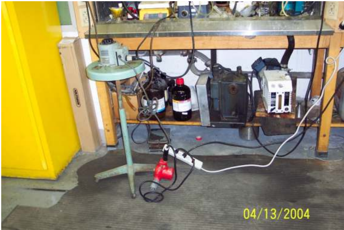
Fig 5.1.1.1: Example of a Potential Accident Area
